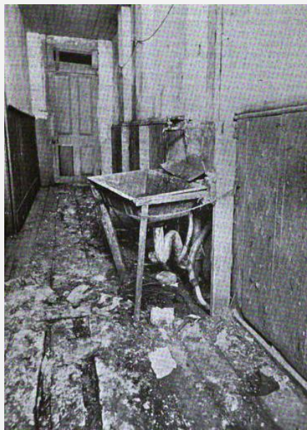
Photo 1.7: Public hall and sink. Sink supported only by string and flimsy wooden props. Hall floor covered with fecal matter and sewage. (1903)
